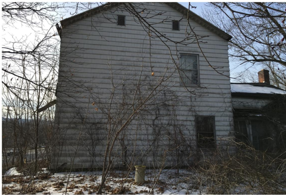
PHOTO VIEW: 2 - East Wall Exterior Elevation
