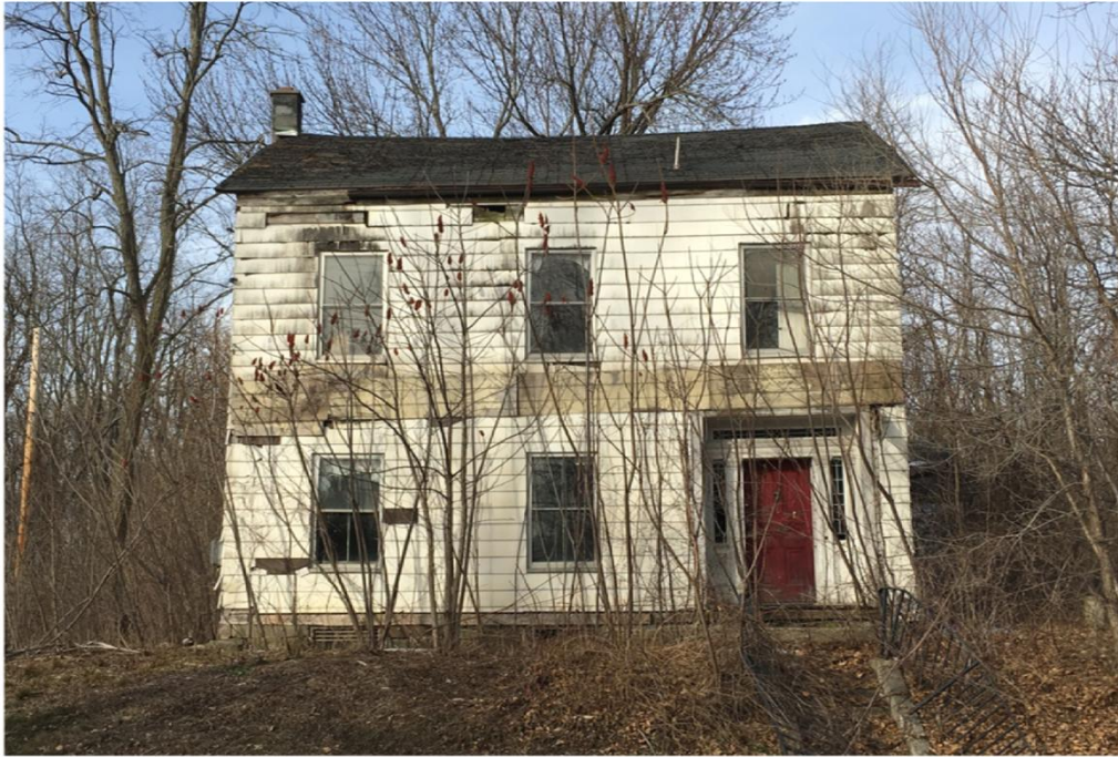
PHOTO VIEW: 1 - South Wall Exterior Elevation - Frontage on State Route 146
