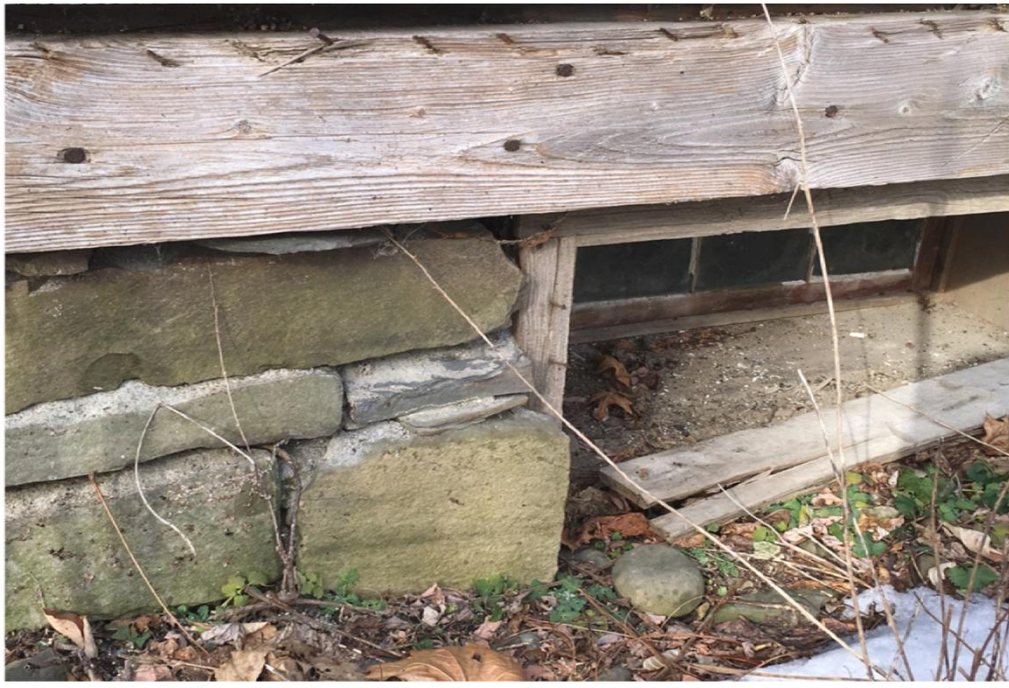
PHOTO VIEW: 5 - Foundation Wall
