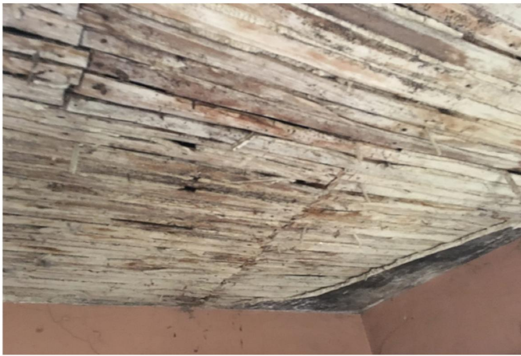
PHOTO VIEW: 12 - Second Floor Bedroom
