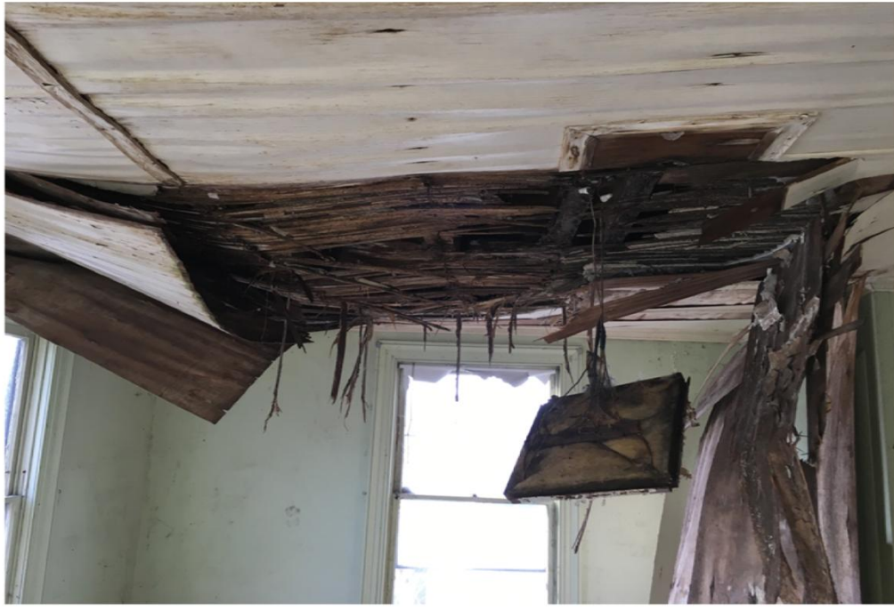
PHOTO VIEW: 11 - Second Floor Bedroom
