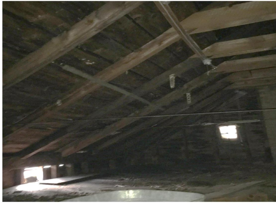
PHOTO VIEW: 13 - Attic Area - Roof Rafters
