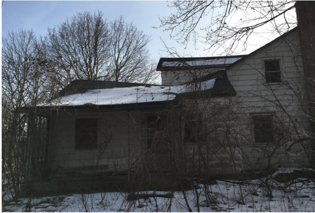
PHOTO VIEW: 3 - North Wall Exterior Elevation
