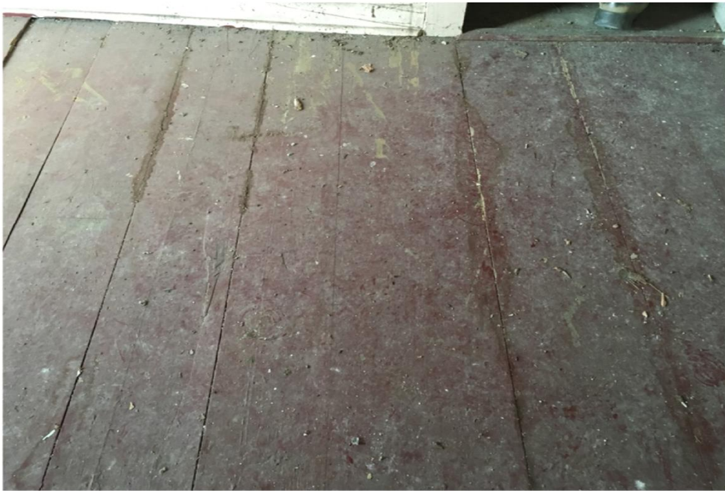
PHOTO VIEW: 10 - Second Floor
