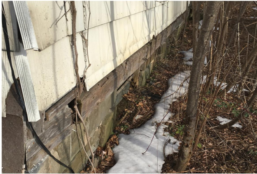
PHOTO VIEW: 6 - Foundation Wall
