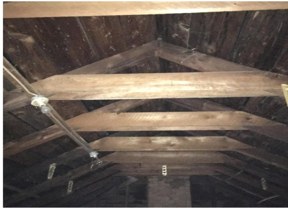
PHOTO VIEW: 14 - Attic Area - Roof Rafters
